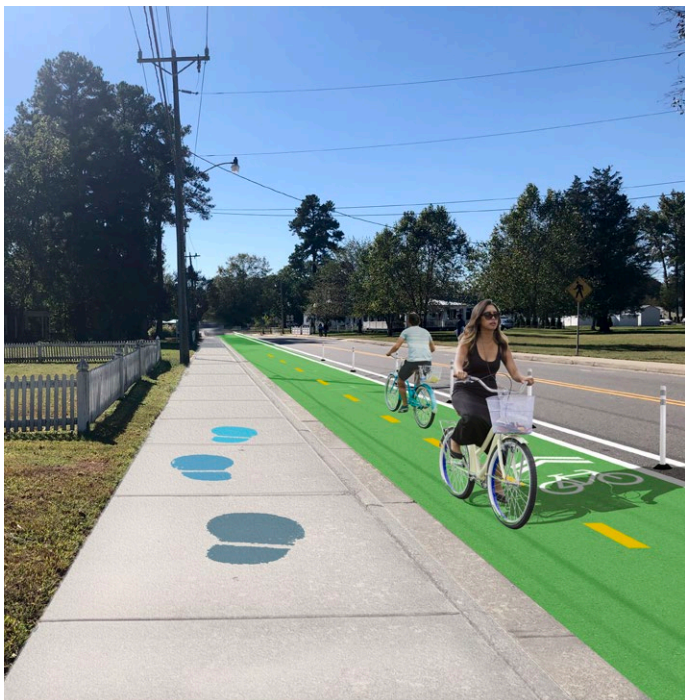
Proposed Condition: Downtown Irvington with dual direction separated bike lanes. 6' sidewalk, 10' bike lane corridor, 2' striped buffer.
