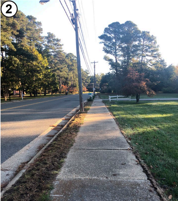
Existing Condition: Irvington Road. 40' curb-to-curb width, 4' sidewalks.
