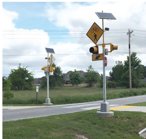
Signaled shared-use path crosswalk
