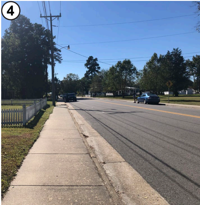
Existing Condition: Downtown Irvington. 40' curb-to-curb width, 4' sidewalks.
